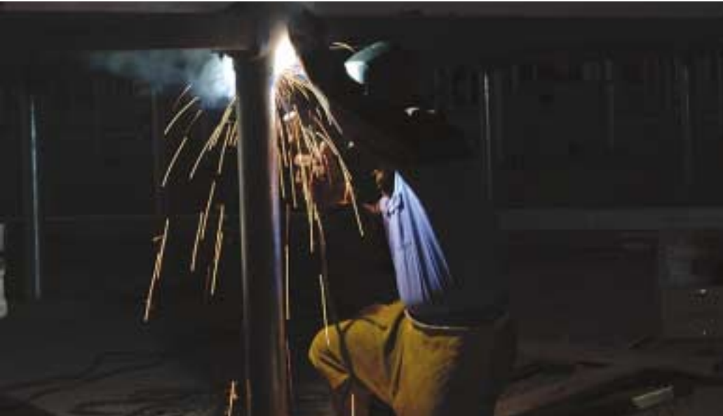
Early morning construction – Chico Water Plant, Ground Mount Tracker 1MW (AC)
