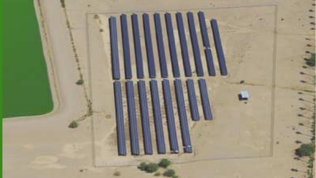
Aerial view of Chuckawalla State Prison, Blythe, CA – 1MW (AC)
